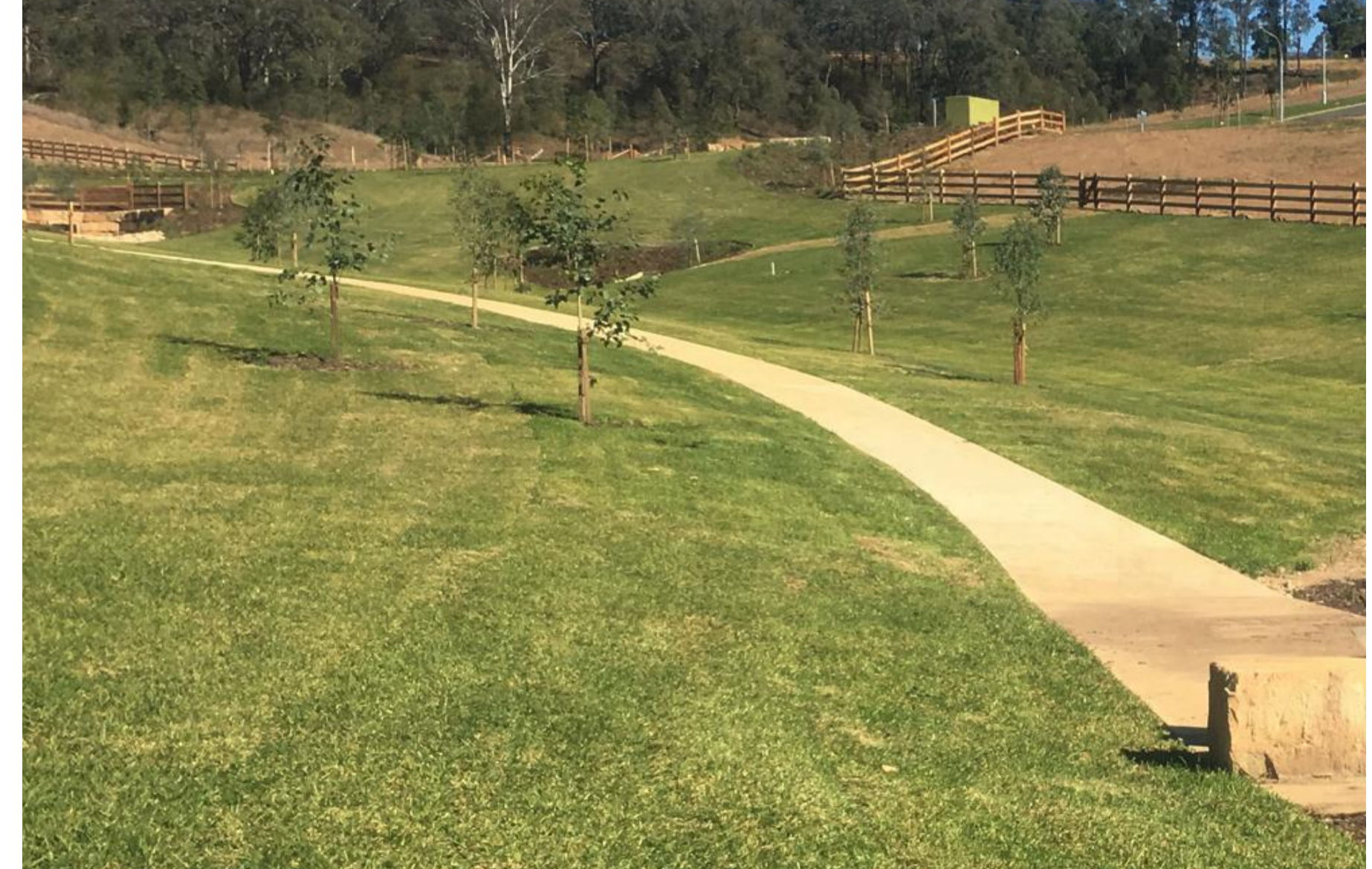
Indicative image of shared concrete pathway and adjoining grass lined swale through open space
